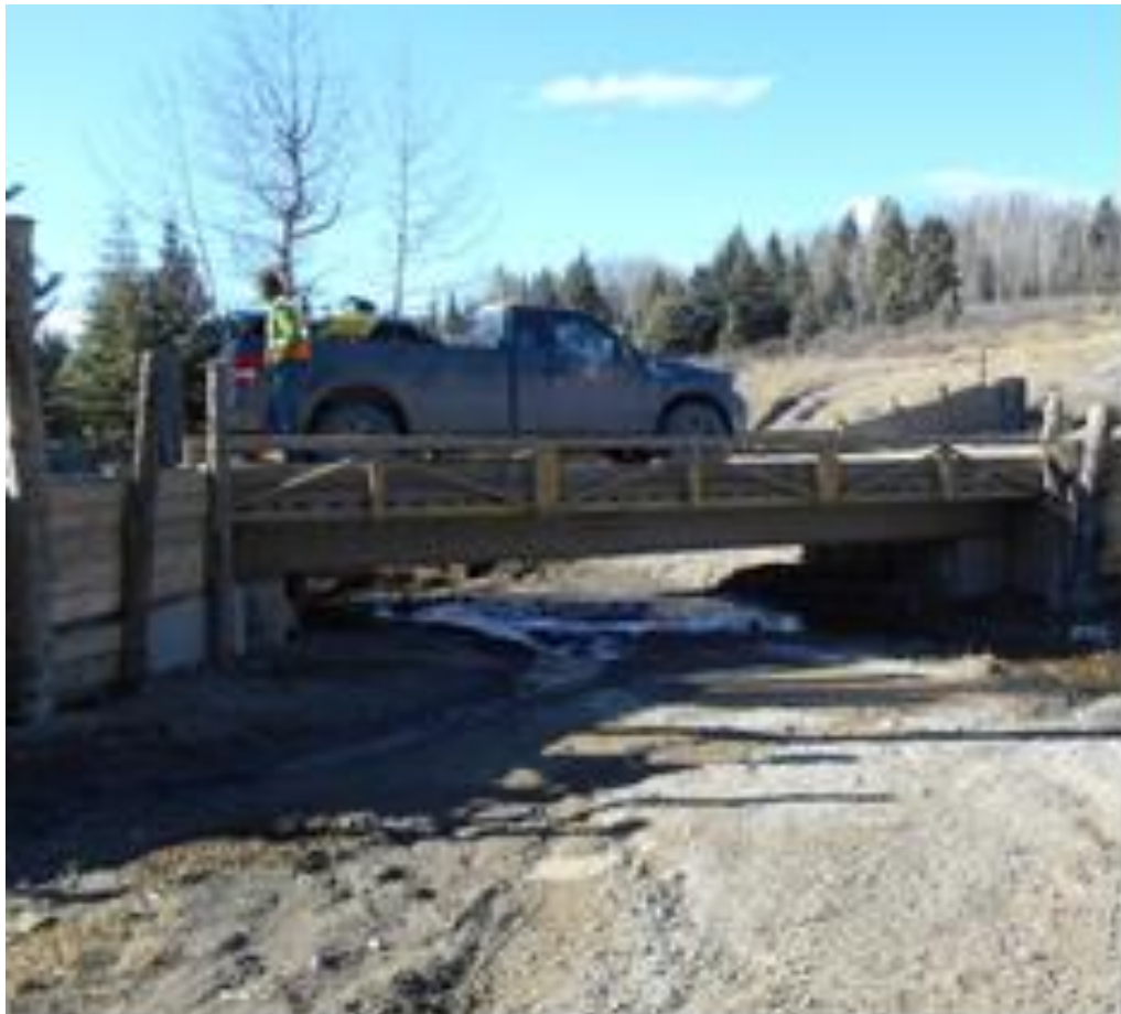
Figure 3. Typical crossing structure on the SLS FMA. Streams are well protected.
